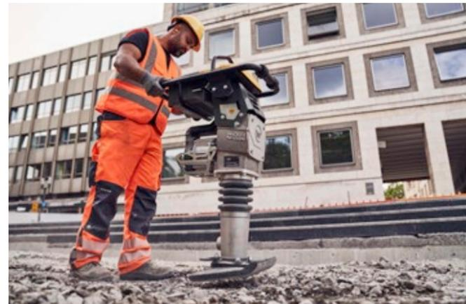
Especially on inner-city construction sites, the battery-powered rammers emit less noise and emissions and thus protect the construction site environment.
