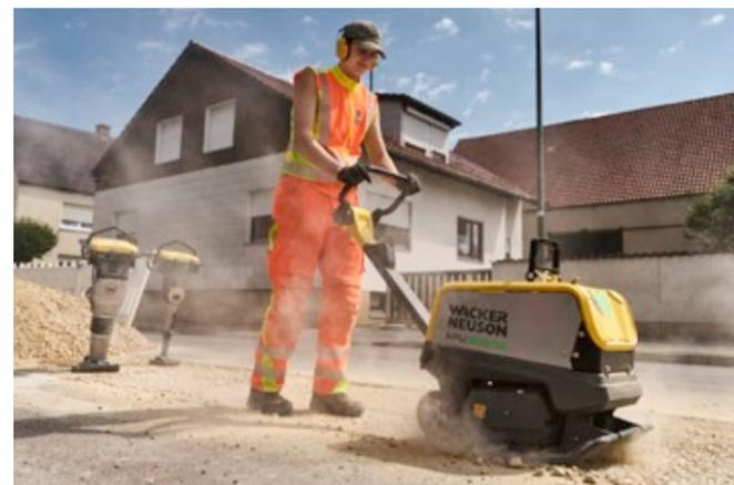
With one battery charge, the APU3050e compacts up to 333 m<sup>2</sup> soil\*.
